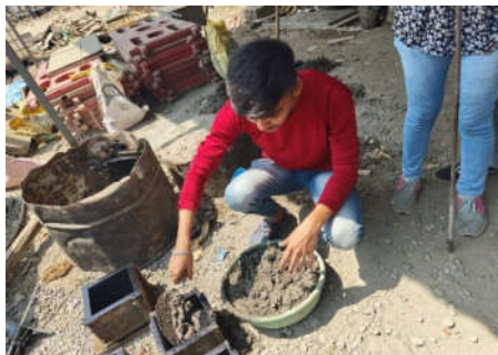
Concrete cube filling
