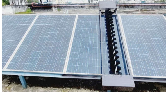
Figure 4 Automated Solar Photovoltaic Panel Cleaning System
