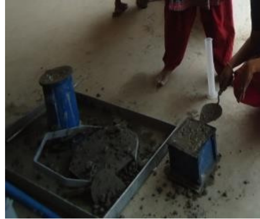
Fig 3.2 Fresh properties of concrete
