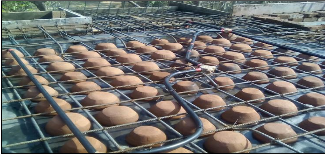
Fig. 8. Roofing with Filler Slab
